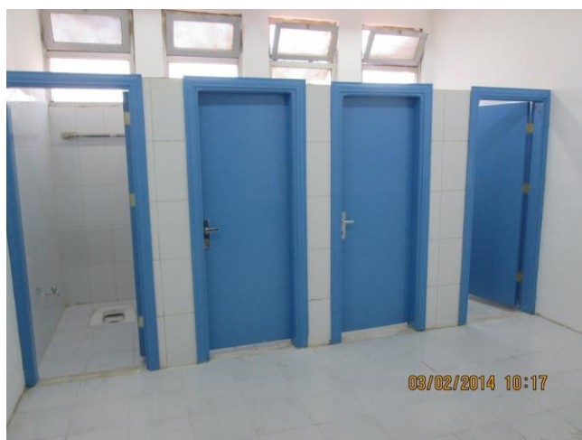
Above: Storage room was converted into new latrines at a Jordanian public school
